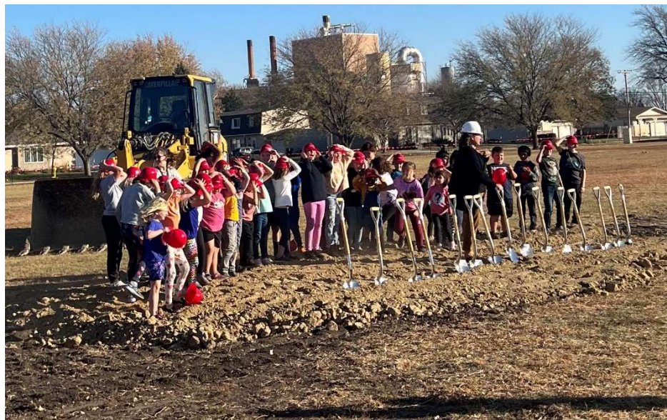
Howard Elementary School students breaking ground at the site of their new elementary school.
